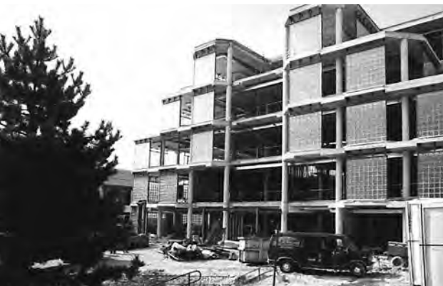
Building construction of the North Campus Library - 1989
