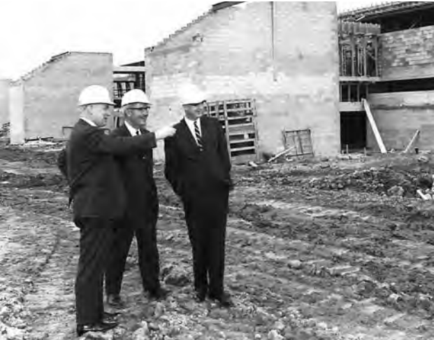
First building construction at the North Campus - 1968
