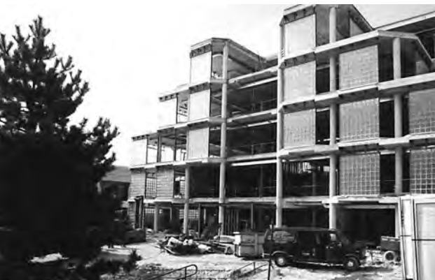
Building construction of the North Campus Library - 1989
