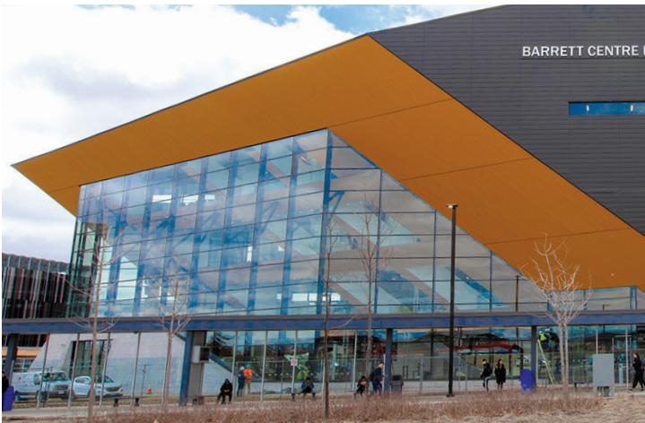
Barrett Centre for Technology Innovation (Barrett CTI), North Campus
