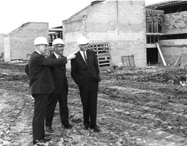
First building construction at the North Campus - 1968
