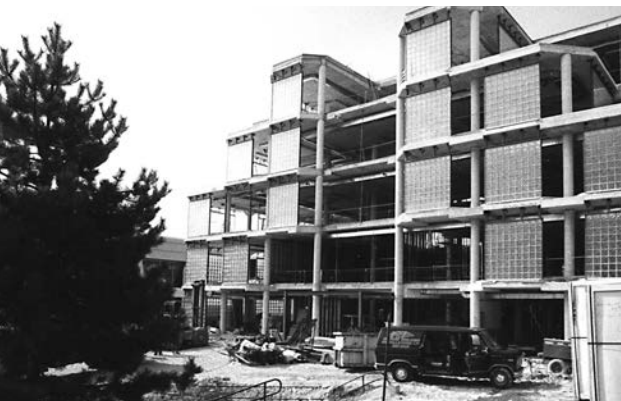
Building construction of the North Campus Library - 1989
