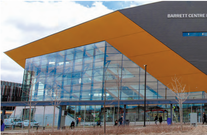
Barrett Centre for Technology Innovation (Barrett CTI), North Campus
