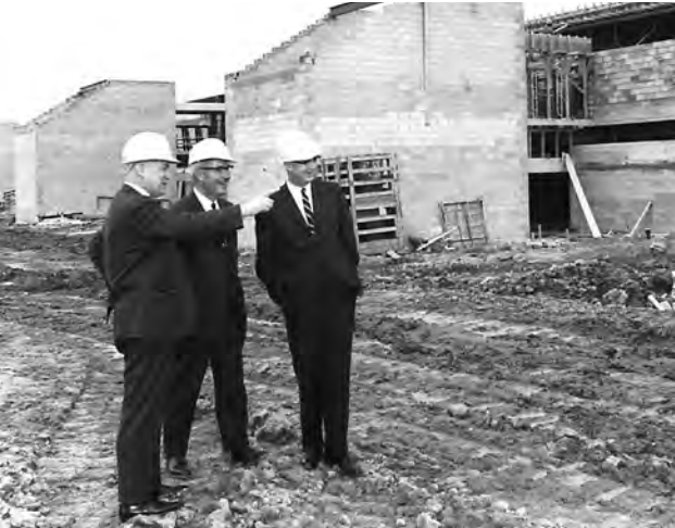
First building construction at the North Campus - 1968
