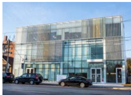
LAKESHORE CAMPUS - FITNESS CENTRE
