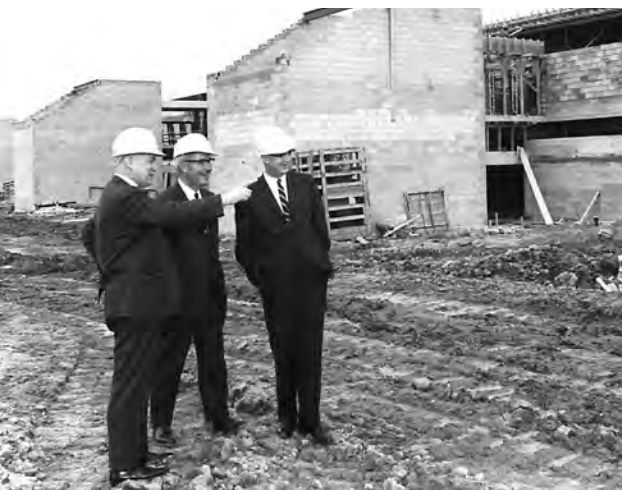
First building construction at the North Campus - 1968
