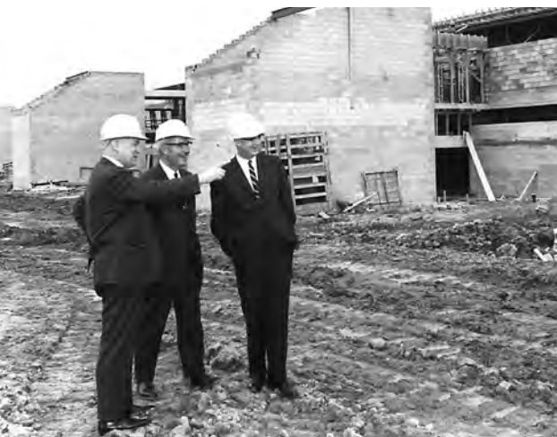
First building construction at the North Campus - 1968
