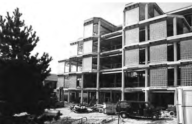
Building construction of the North Campus Library - 1989
