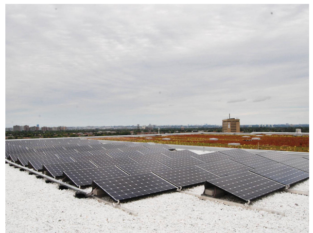
Above: Solar panels and green roof of the LRC
